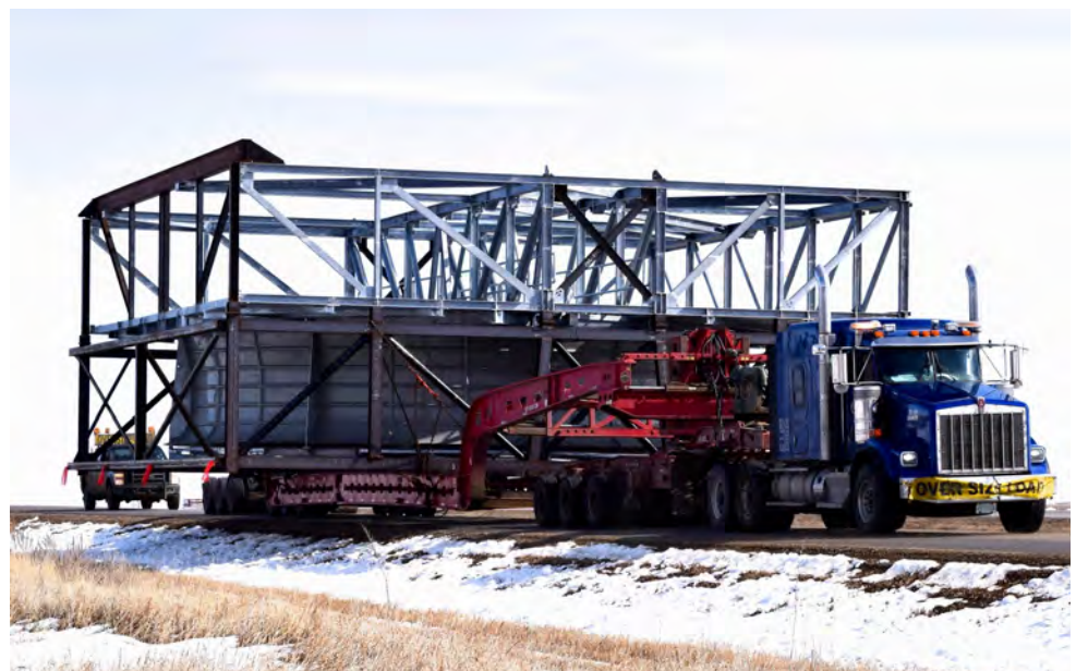
This module was designed with supports for transportation. The darker steel will be removed prior to installation on-site.
